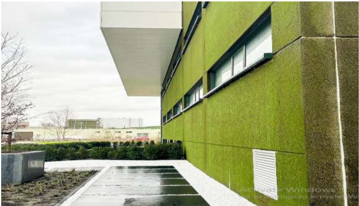
Figure 30: Application of Moss Concrete by Respyre, Netherlands.
