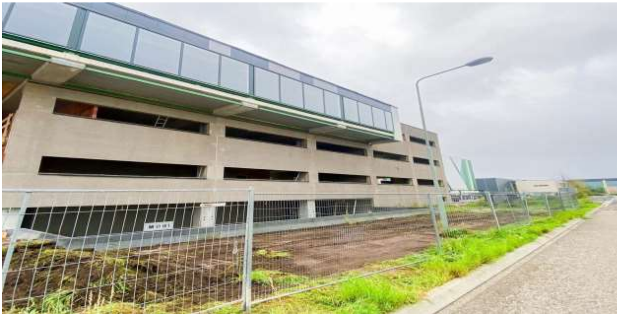
Figure 28: Before the application of Moss Concrete. An Office cum Warehouse Building, Hoex Bouw and Schelfhout Belgium Carrelages - Tegels.
