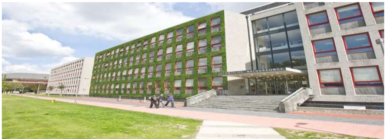
Figure 26: Application of Moss Concrete. TU Delft Campus Building by Respyre.
