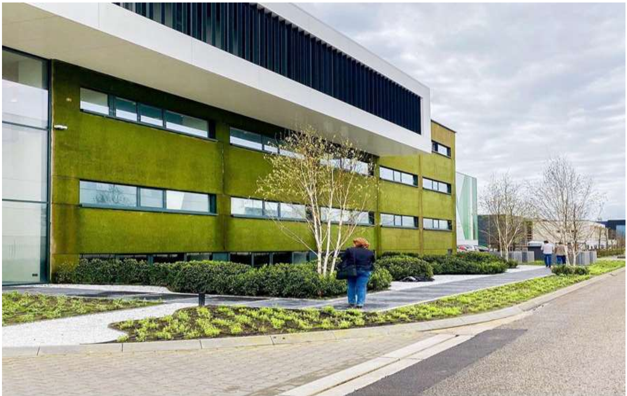
Figure 29: After the application of Moss Concrete. An Office cum Warehouse Building, Hoex Bouw and Schelfhout Belgium Carrelages - Tegels.
